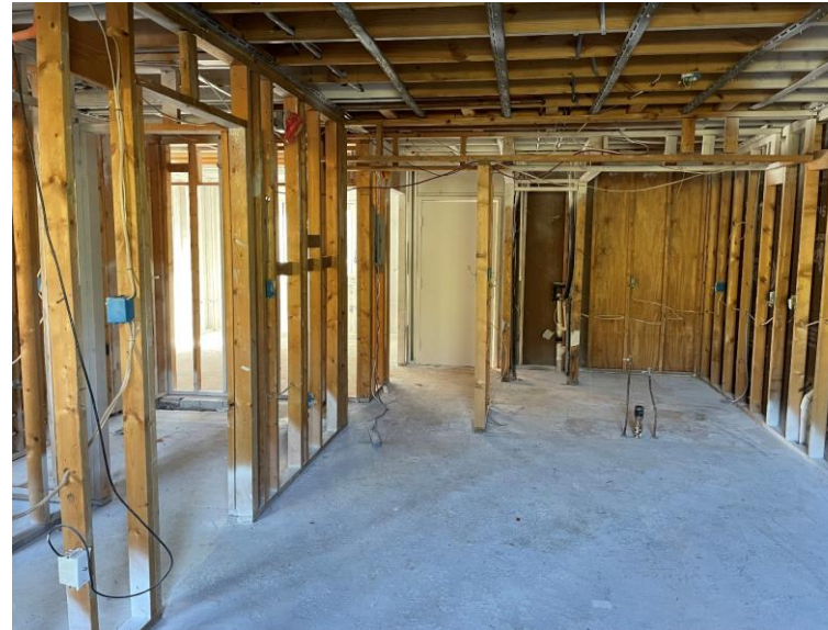
Gutted interior after water-damaged gypsum wallboard and finishes removed
