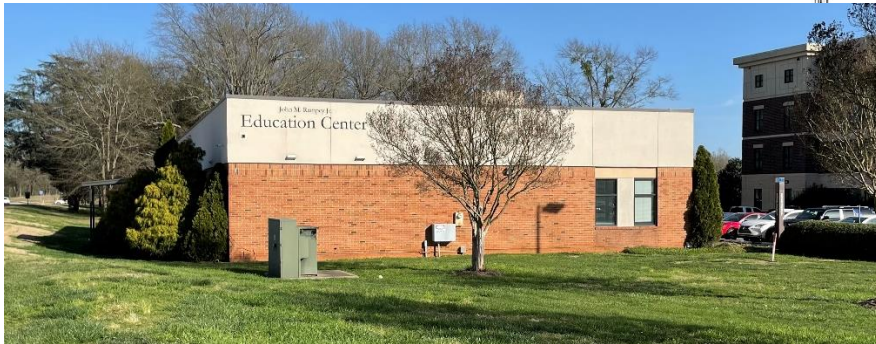
Exterior and area of expansion
